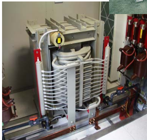
Water-cooled DC link Reactor
