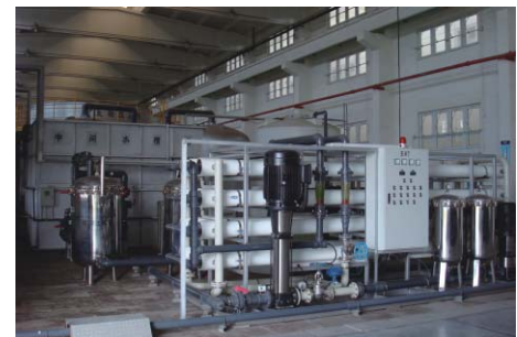
Sewage treatment system
