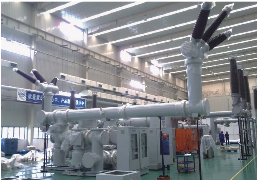
Kiev Boryspil International Airport-126kV GIS The Ukrainian Kiev Boryspil International Airport Project is one of the important projects from the 2012 European Cup.
