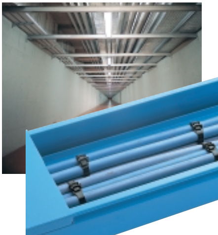
Fixing cables in ducts and/or raceways.
