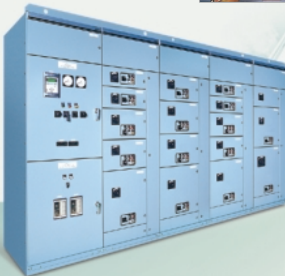
Low Voltage Switchboard System
