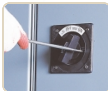
Operating handle is interlocked with door for basic safety. Screwdriver-operated defeater is provided. Door cannot be opened with circuit breaker ON, nor can circuit breaker be turned ON with door open, unless the defeater is used.
