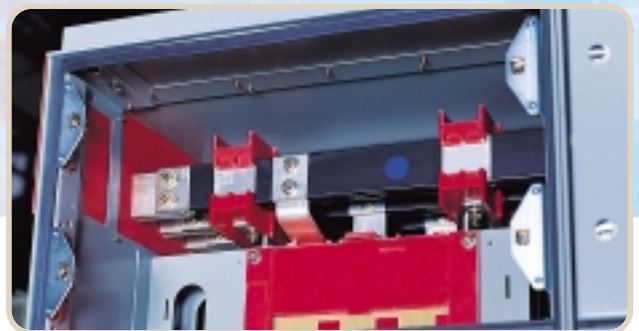
All bus bar joints are made with bolts with washers to ensure permanent tightness.
