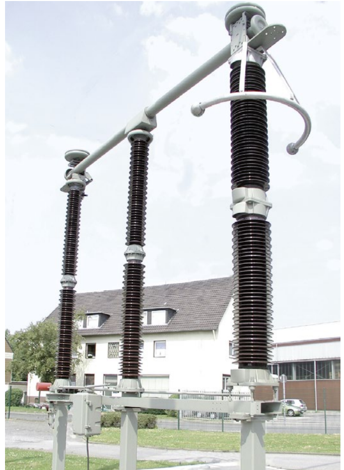
Fig. 4.2-5: Double-side break disconnector with integrated surge arrester
