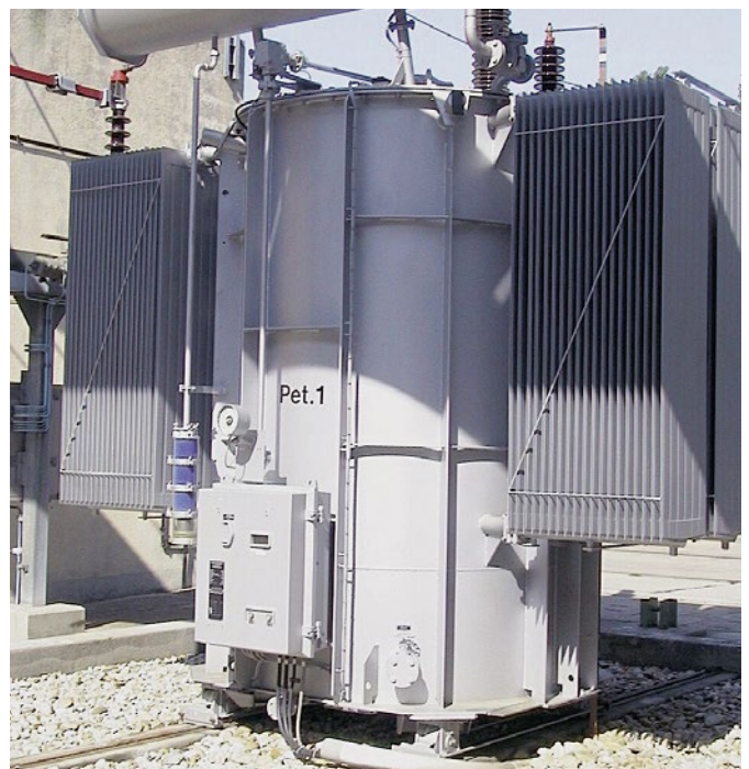
Fig. 4.7-5: Arc-suppression coil 110 kV
