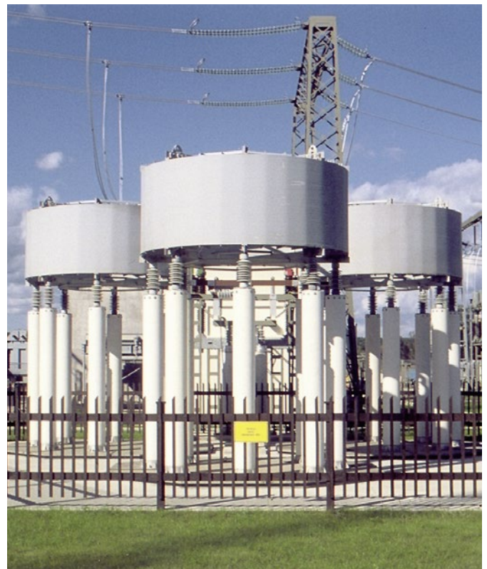
Fig. 4.7-3: Tertiary-connected shunt reactors
