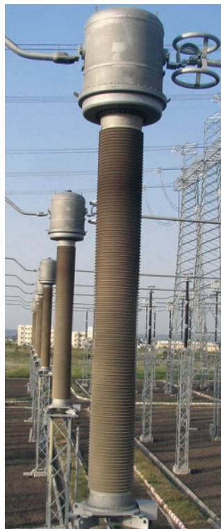
Fig. 4.6-1: 800 kV gas-insulated current transformers
