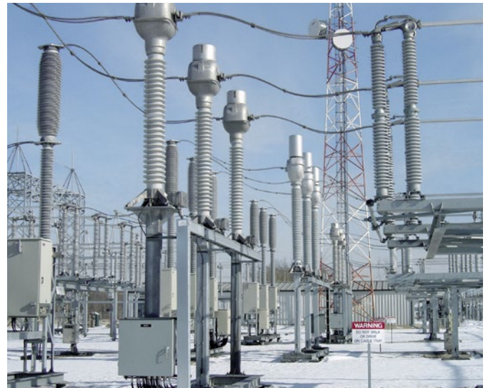
Fig. 4.6-3: 300 kV oil-immersed current transformers
