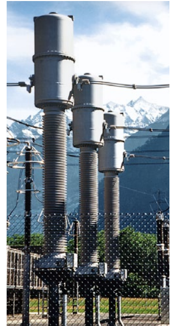
Fig. 4.6-9: 420 kV gas-insulated combined instrument transformers
