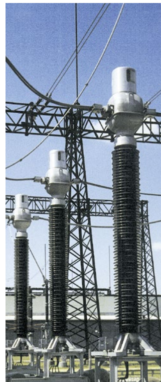
Fig. 4.6-2: 550 kV oil-immersed current transformers
