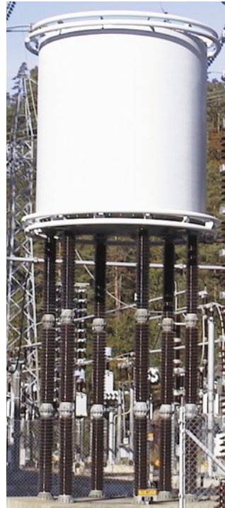
Fig. 4.7-4: HVDC smoothing reactor
