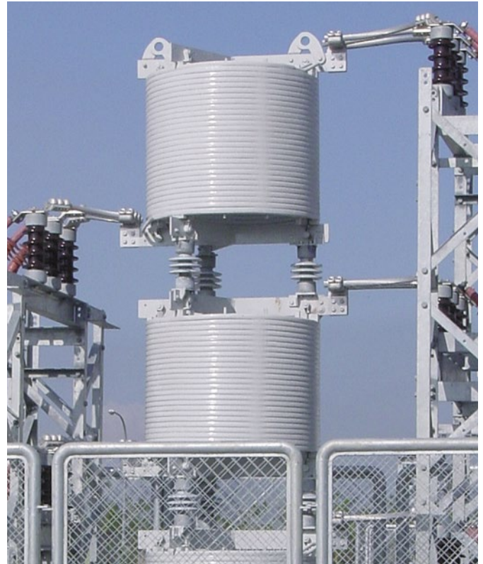
Fig. 4.7-2: 3-phase stacked current-limiting reactor
