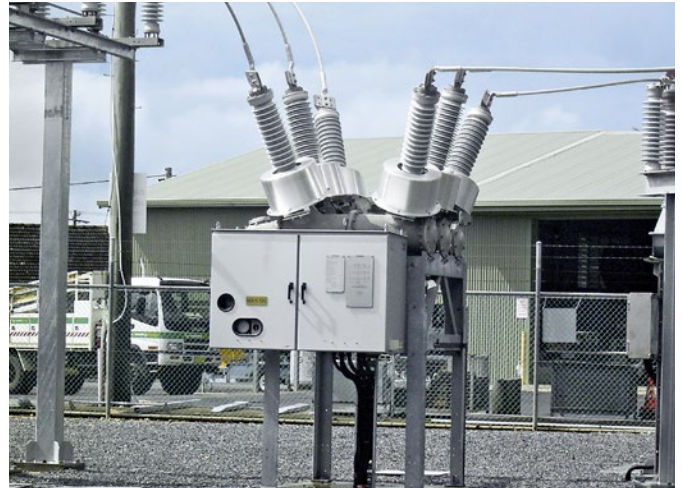
Fig. 4.1-11: SPS2/3AP1 DT 72.5 kV
