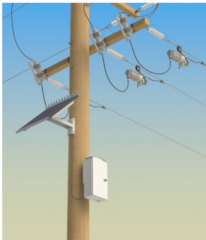
Fig. 4.3-10: Fusesaver and RCU installation (with solar panel for RCU)
