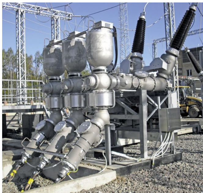
Fig. 4.1-20: 3AP1 DTC 145 kV with voltage transformer and cable connection
