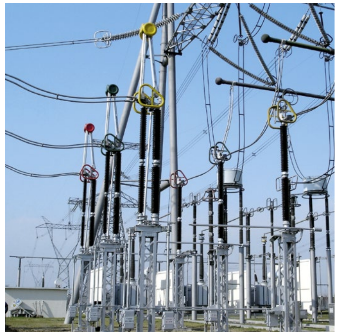
Fig. 4.2-6: Knee-type disconnector
