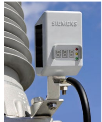
Fig. 4.5-6: Arrester condition monitor (ACM)
