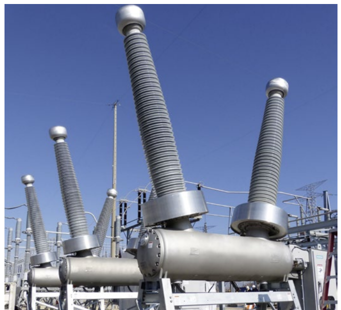
Fig. 4.1-13: SPS2/3AP1 DT 362 kV (two-cycles)
