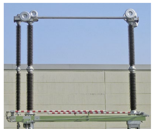
Fig. 4.2-4: Vertical-break disconnector
