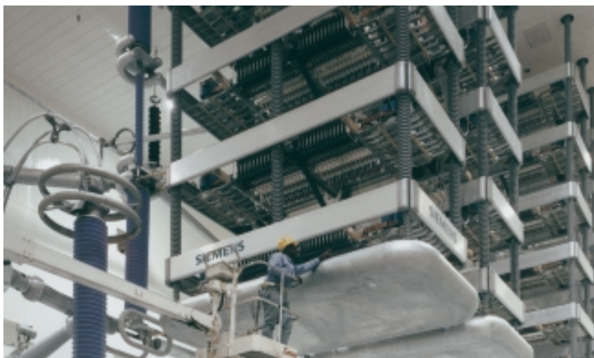
Fig. 76: Earthquake-proof, fire-retardant thyristor valves in Sylmar East, Los Angeles
