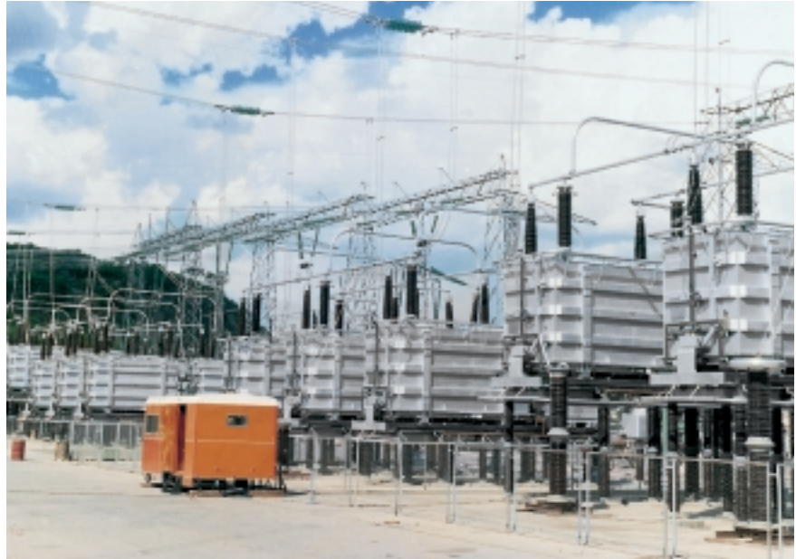
Fig. 78: HVDC outdoor valves, 533 kV (Cahora Bassa Rehabilitation, Southern Africa)
