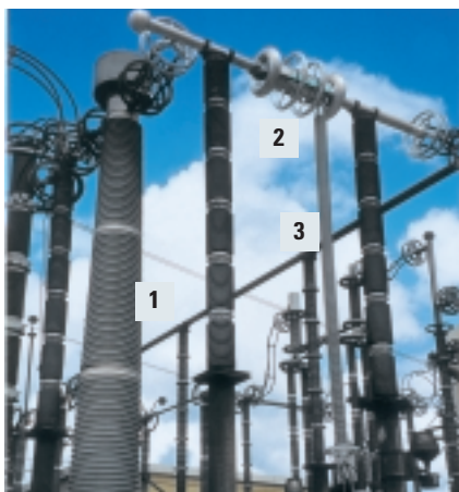
Fig. 77: Conventional DC measuring device (1) vs. the new hybrid-optical device (2) with composite insulator (3) shows the reduced space requirement for the new system (installed at HVDC converter station Sylmar, USA)
