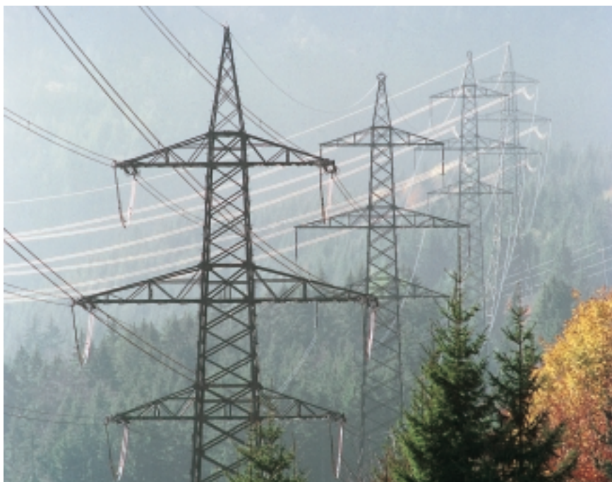
Fig. 69: Lattice steel towers of a high-voltage line
