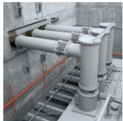
Fig. 55: Transformer termination modules
