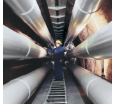
Fig. 57: GIL arrangement in the tunnel of the Wehr pumped storage station (4000 m length, in service since 1975)
