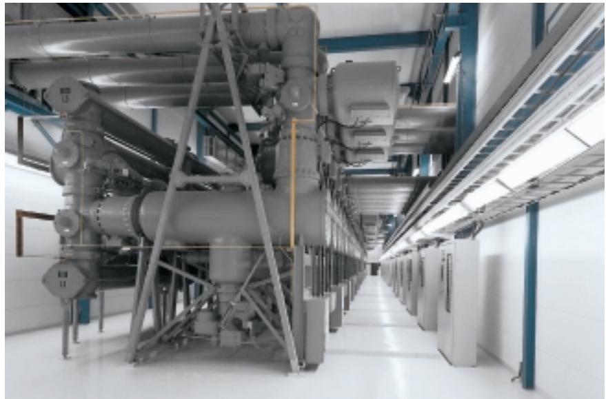
Fig. 47: 8DQ1 switchgear for rated voltage 420 kV
