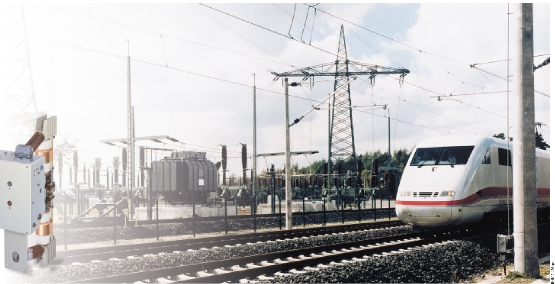
Körle substation, 110 / 15 kV, 16 2 / 3 Hz (traction power supply) with ICE power unit
