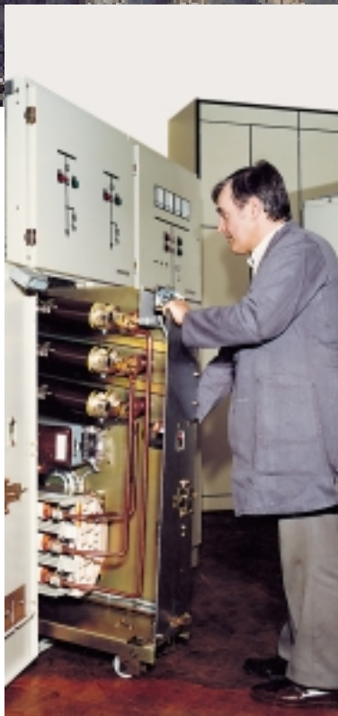
Siemens 8BK30 medium-voltage withdrawable switchgear with 3TL6 vacuum contactor on central truck
