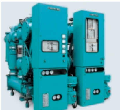
Fig. 2a: Protection and control in HV GIS switchgear
