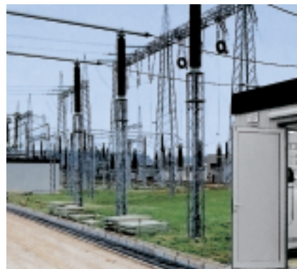
Fig. 2b: Protection and control in bay dedicated kiosks of an EHV switchyard
