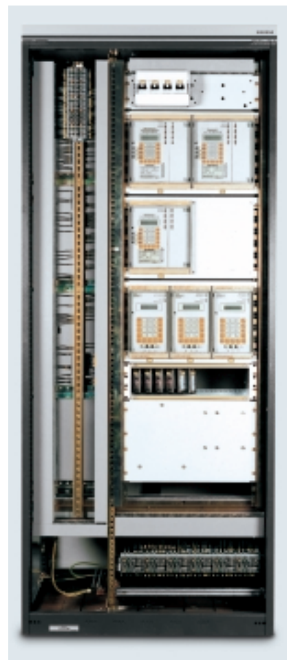
Fig. 65b: Numerical protection of a generating unit (example). Cubicle design.
