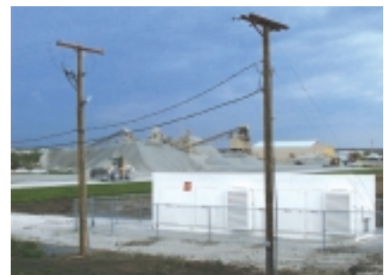
Fig. 254: Active compensation system (Power Conditioner DSTATCOM)
