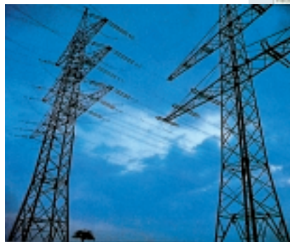
Fig. 246: ... and to monitor transmission lines
