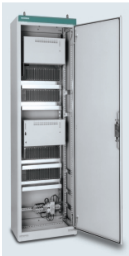
Fig. 169: SINAUT LSA COMPACT 6MB5540 remote terminal unit installed in a cubicle
