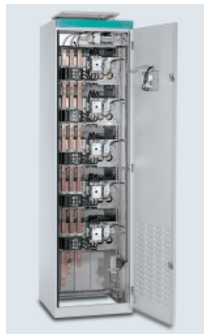
Fig. 271: 4RF1 power factor correction unit 250 kvar (5 x 50 kvar) in a cabinet 2275 x 625 mm
