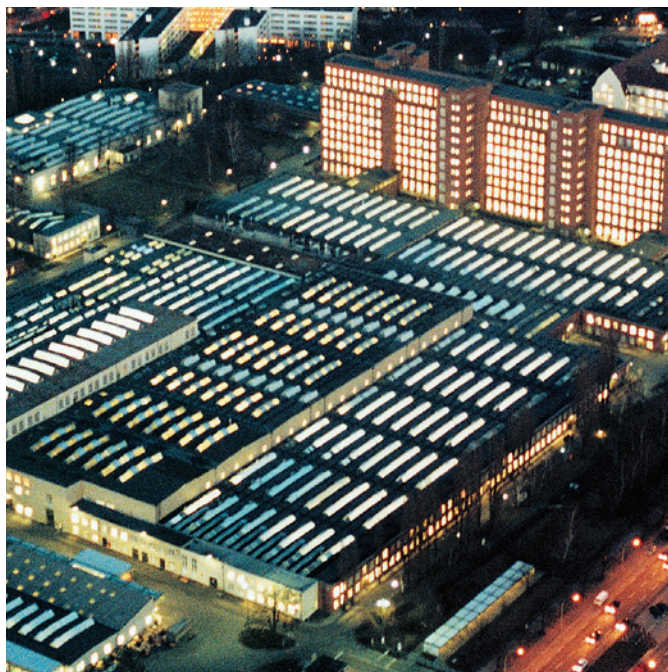
Switchgear Factory in Berlin, Germany
