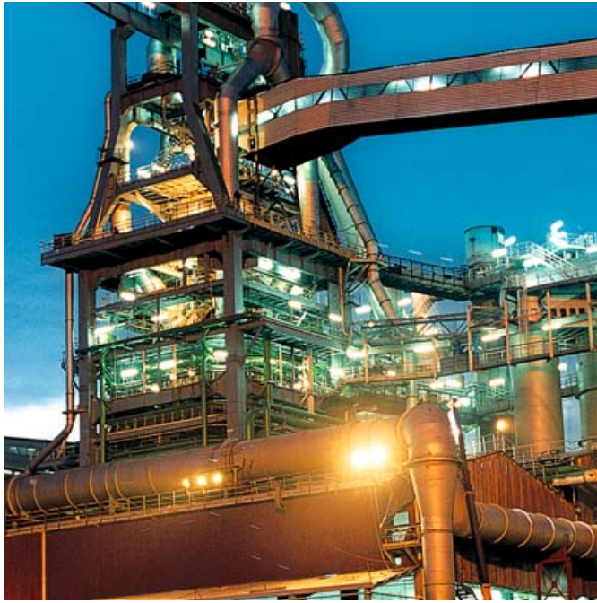
Industrial application: Refinery
