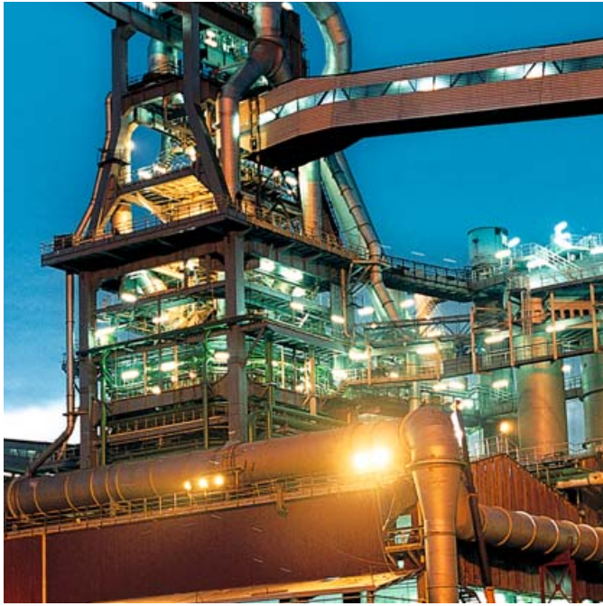
Industrial application: Refinery
