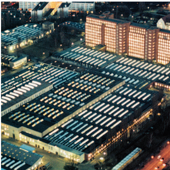
Switchgear Factory in Berlin, Germany
