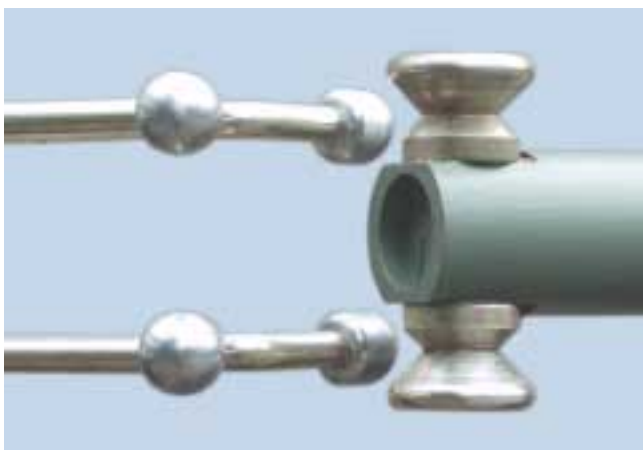
Opening main contacts of a centre break disconnector
