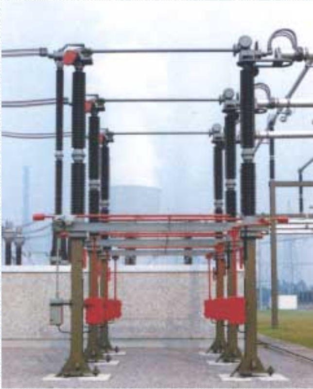
Vertical break disconnector, ON position
