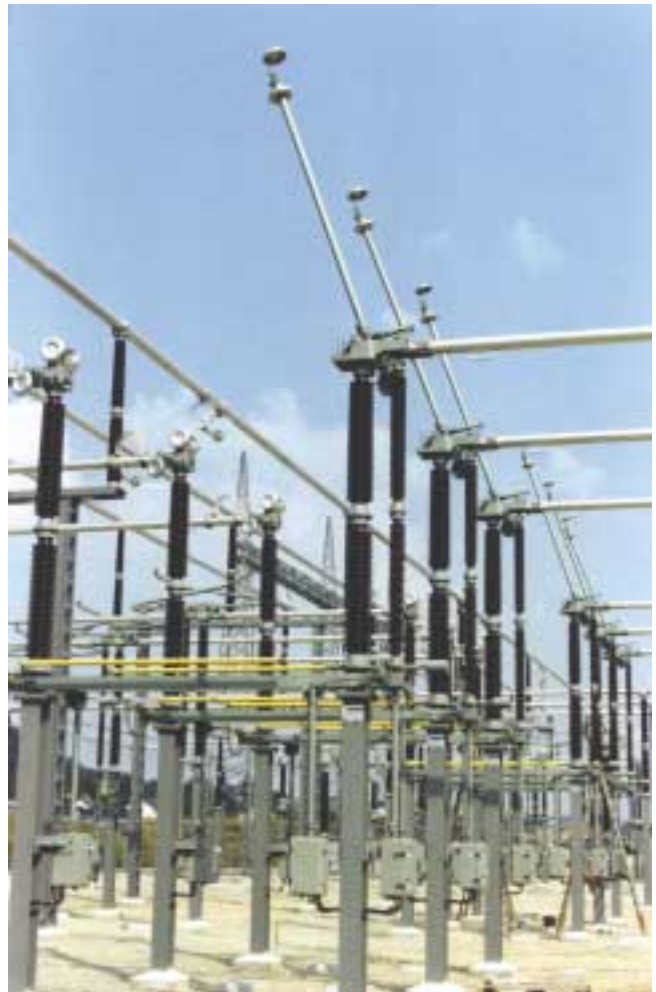
Vertical break disconnector, OFF position
