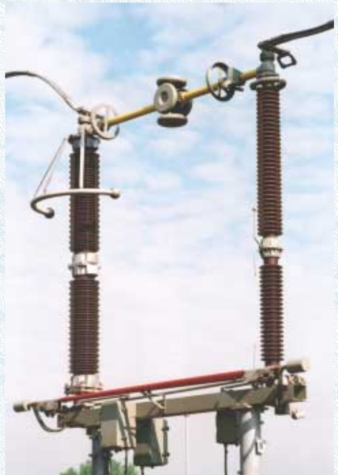
Centre break disconnector with integrated surge arrester
