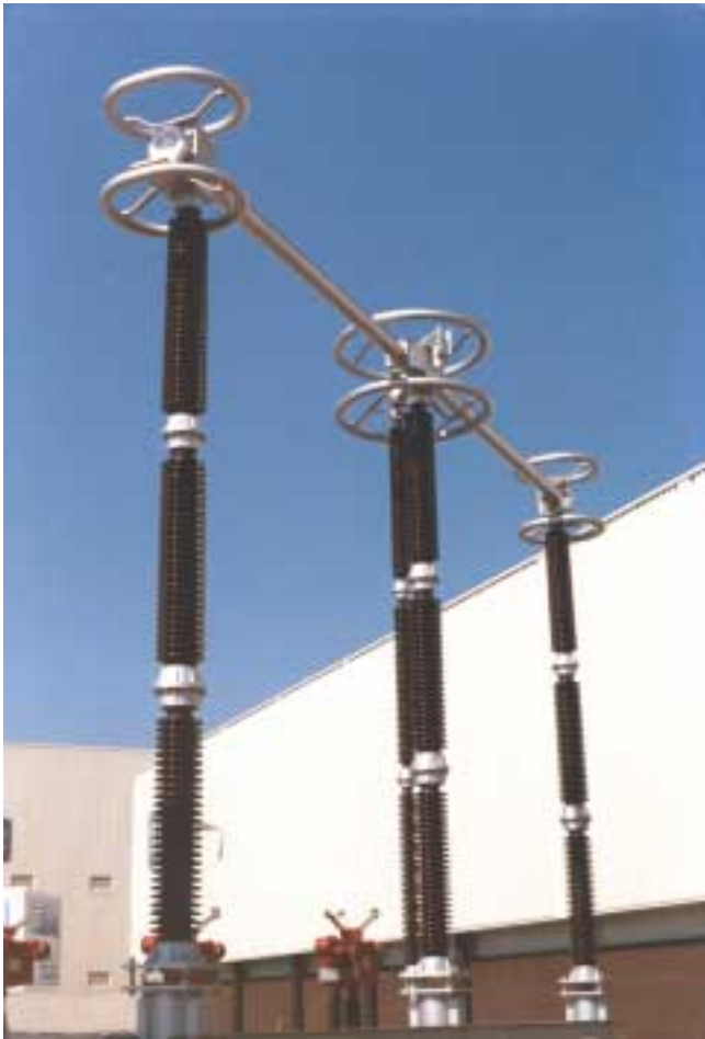
Double side break disconnector, special design for 800 kV
