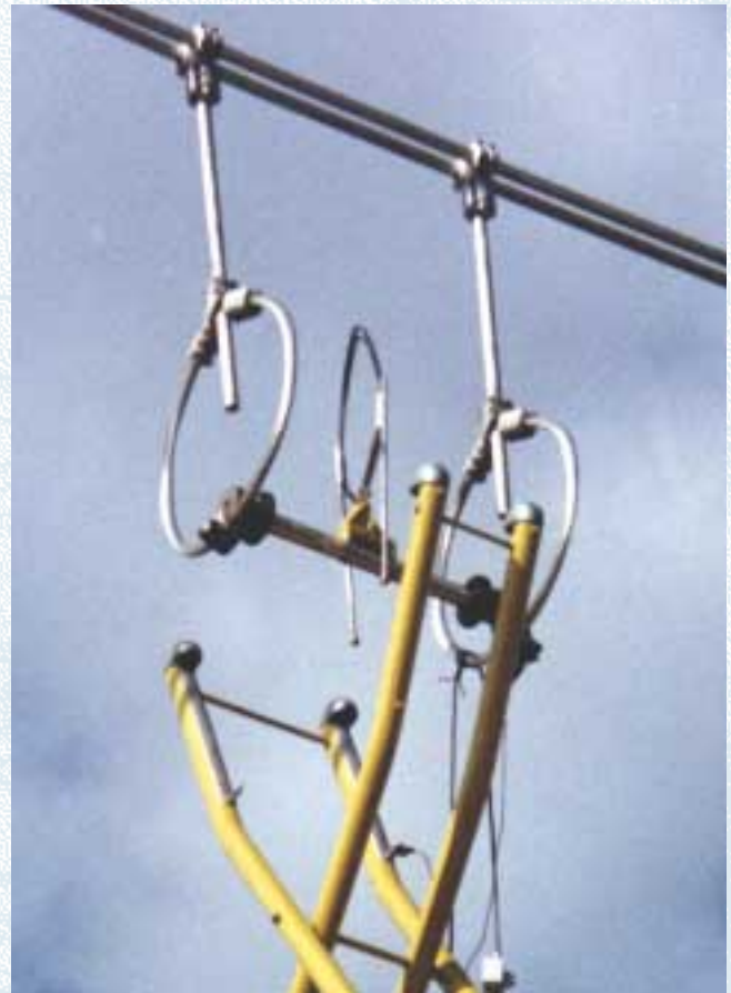
Contact system of a pantograph disconnector with commutating contacts
