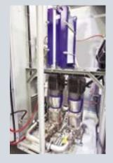
Integral Water to Water Heat Exchanger
