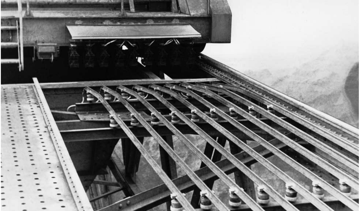
Bridge Crane Conductor Transfer Ends
